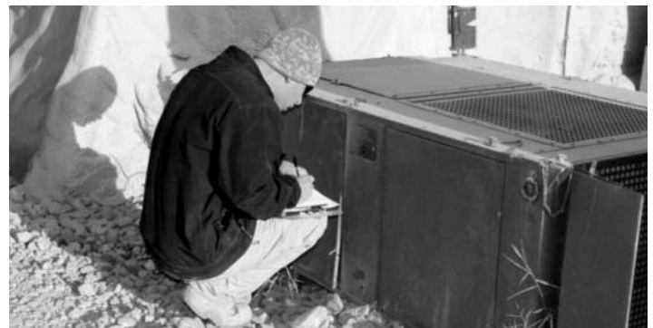
Figure 1. Chris setting up HVAC system.
